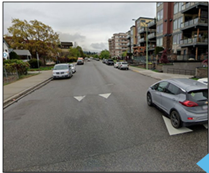
A speed table is like a speed hump, but long enough to raise the entire wheelbase of a car and has a flat top. Their aim is to slow down traffic speeds. Sometimes they are designed as raised midblock crossings with curb extensions.
