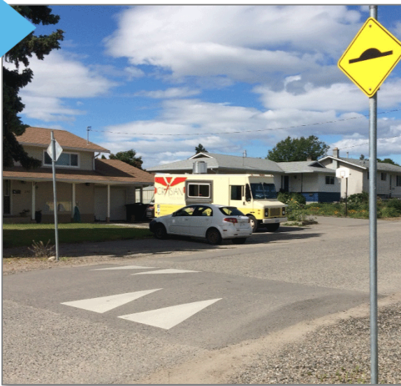
A speed hump is a raised area of the roadway that slows down traffic speeds. It is a cost effective and commonly used traffic calming measure.
